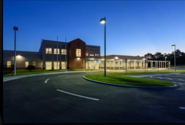
HIDDEN OAKS ELEMENTARY SCHOOL
