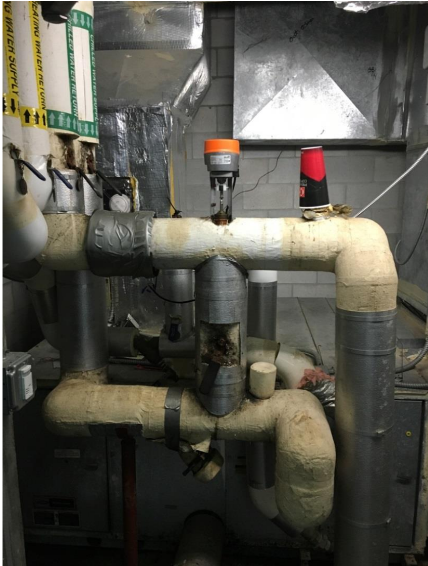
Aged heating and air-conditioning units and miscellaneous “fixes” for obsolete components.
