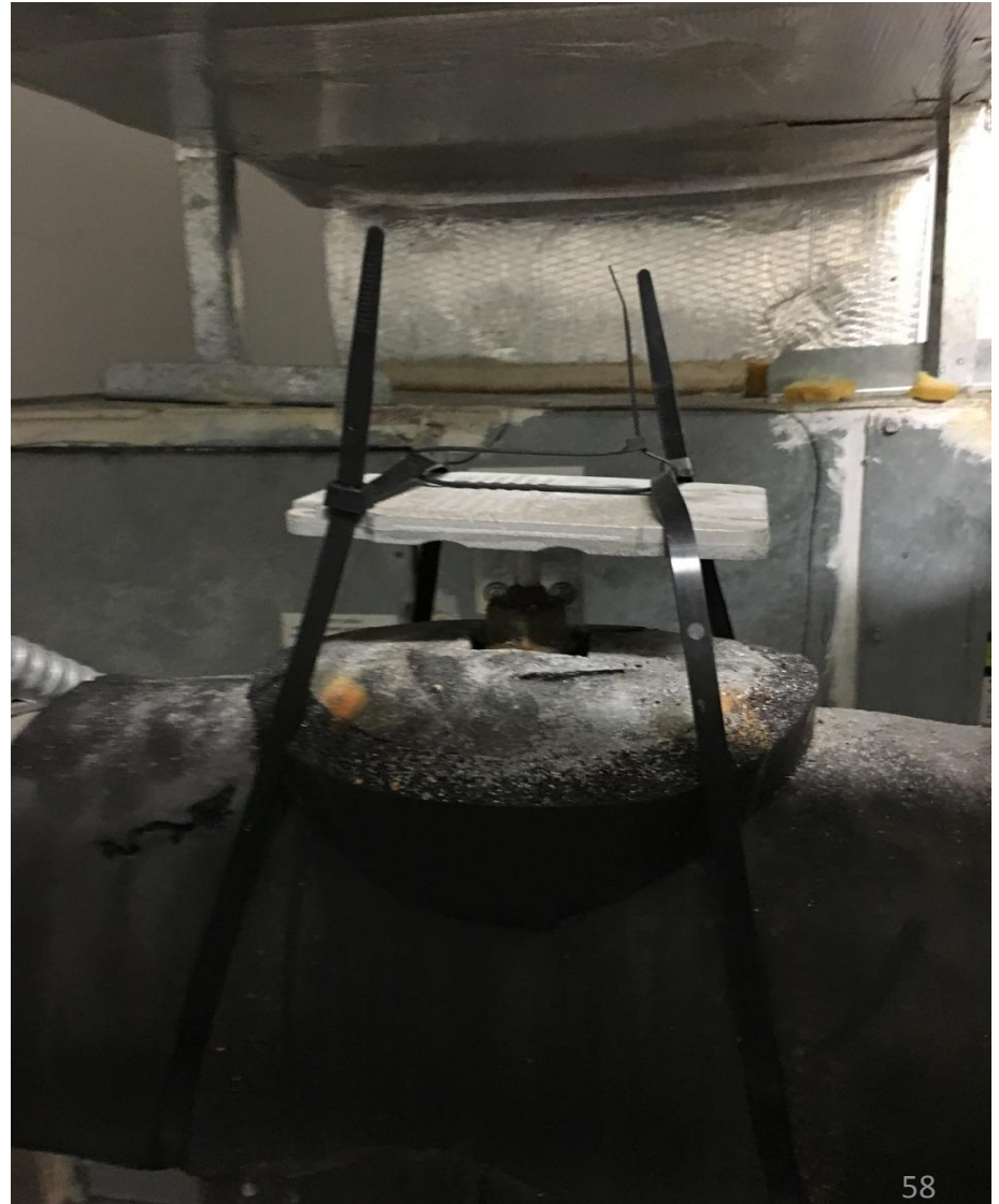
Aged heating and air-conditioning units and miscellaneous “fixes” for obsolete components.
